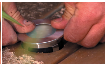
COMPLETE INSTALLATION OF LIGHTS
