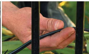
RUN LOW VOLTAGE CABLE
