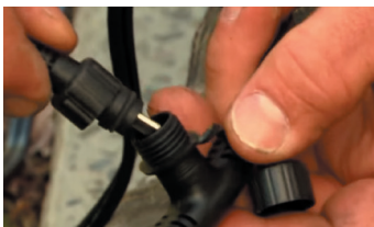
PLUG YOUR LIGHTS INTO THE CABLES
