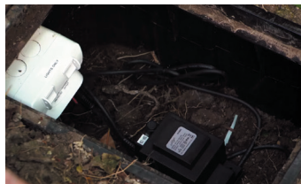
POSITION YOUR LOW VOLTAGE TRANSFORMER
